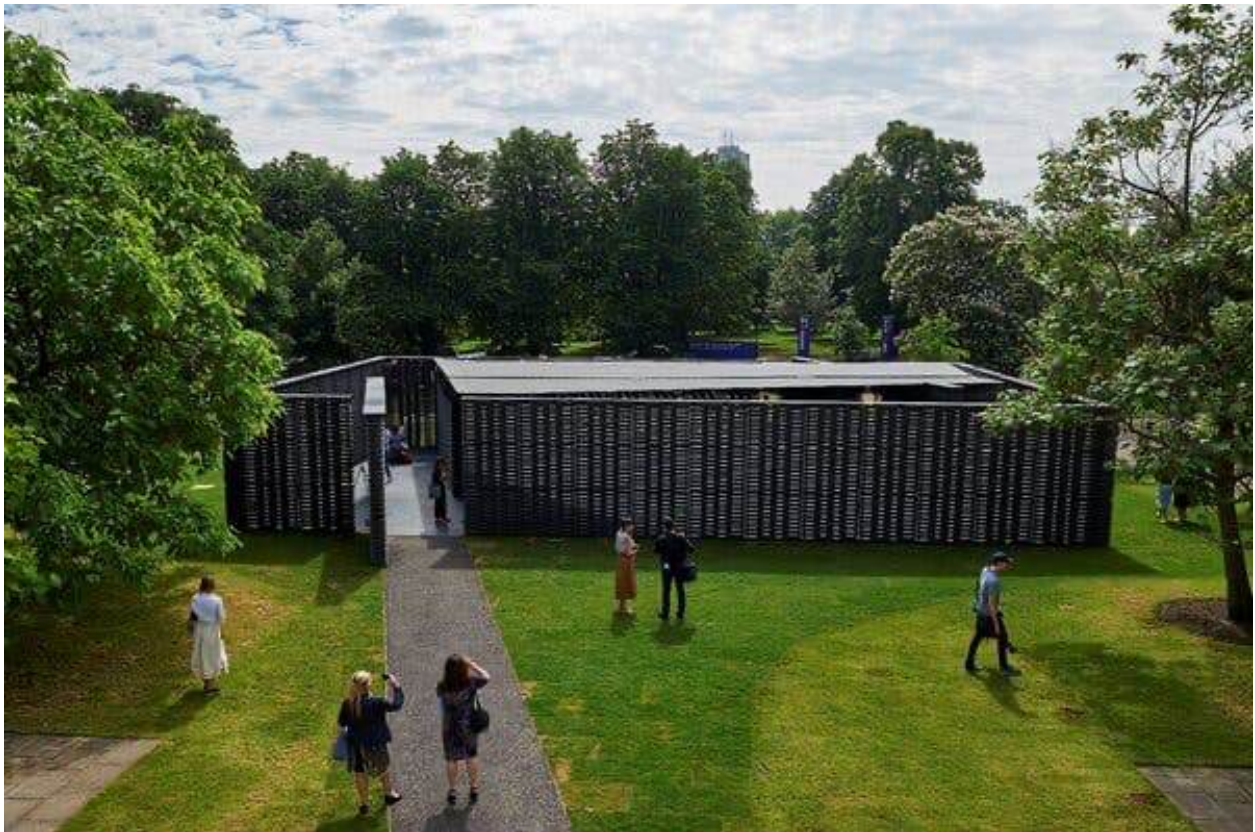
For the Serpentine Pavilion in London, in 2018, Escobedo reinterpreted Mexican elements to create a perforated wall of concrete roofing tiles. Credit...Niklas Halle'N/Agence France-Presse — Getty Images
