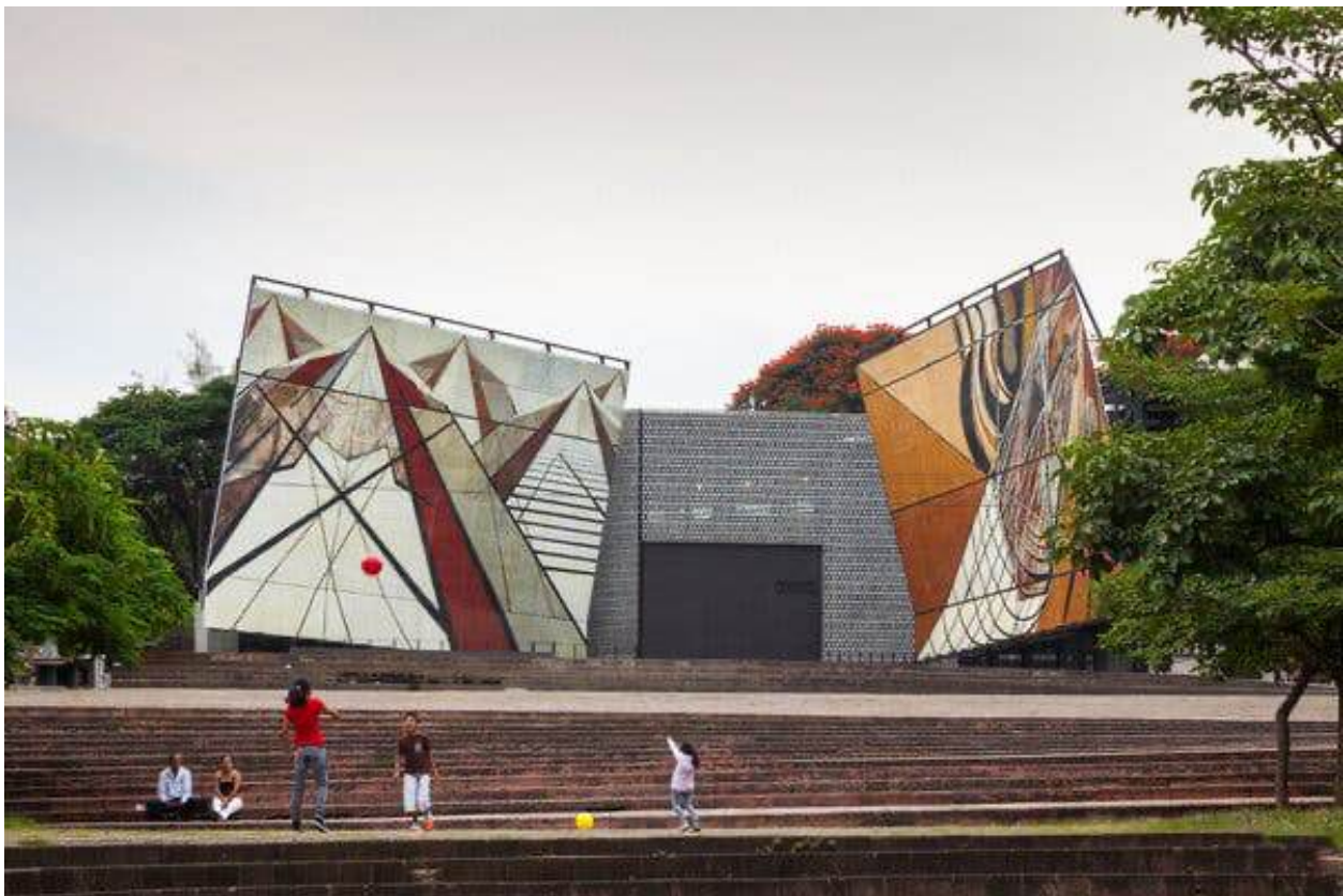
The Escobedo-designed expansion of La Tallera Siqueiros, a museum, workshop and artist’s residence in Cuernavaca, Mexico. The architect opened the museum’s courtyard to the plaza by rotating murals by David Alfaro Siqueiros from their original position, making them part of the facade. Credit...via Frida Escobedo Studio; Photo by Rafael Gamó
