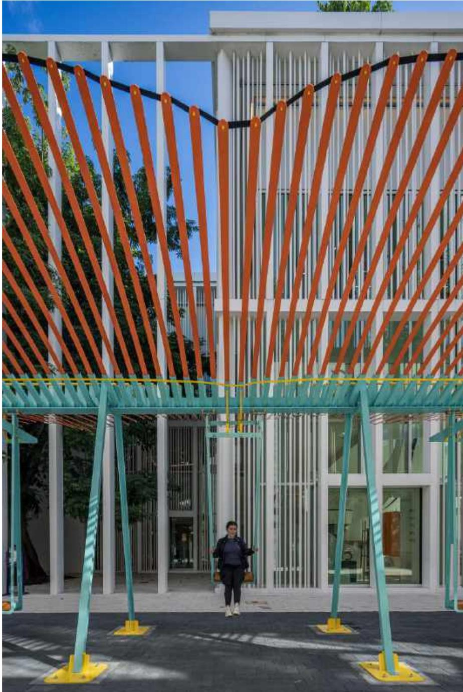
Elastic connects the slats triggering the ripples
